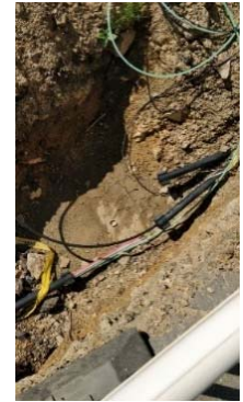
Fiber optic cable laying in a village (Source: K. Illigmann)
